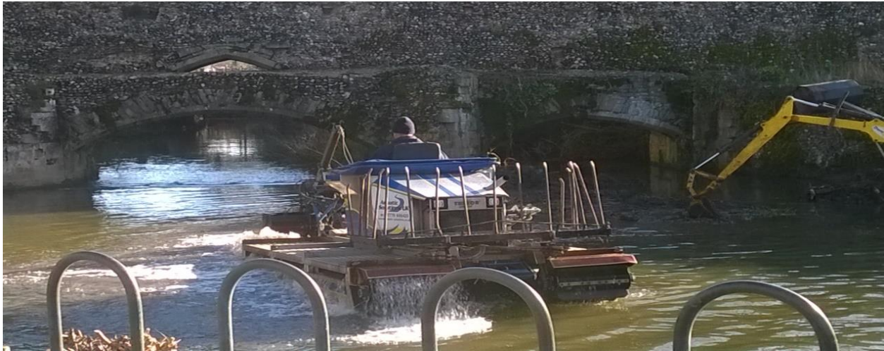
River Lark Restoration near the Abbey Gardens, Bury St Edmunds
